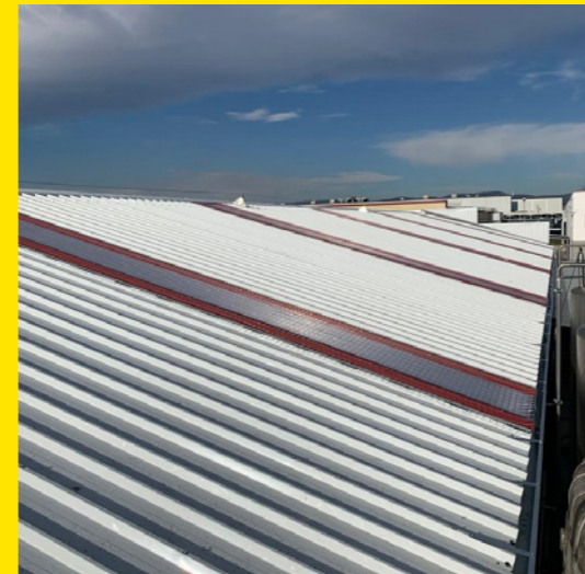
Moving forward on the green electricity transition.
